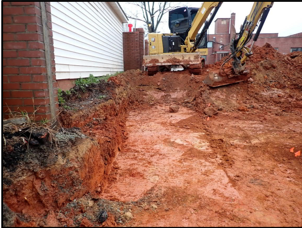
Figure 4. General Overview of Soil Profile (at left) with Fill and Underlying Red Clay Subsoil, View North.
